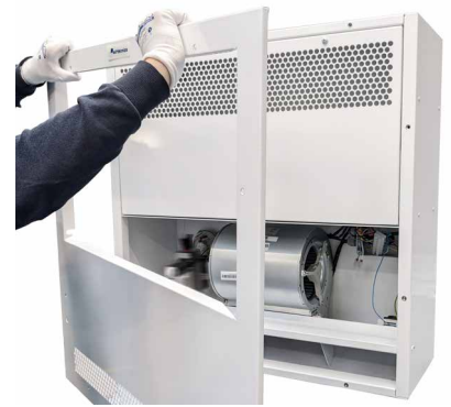
2- Gently remove the service panel down
