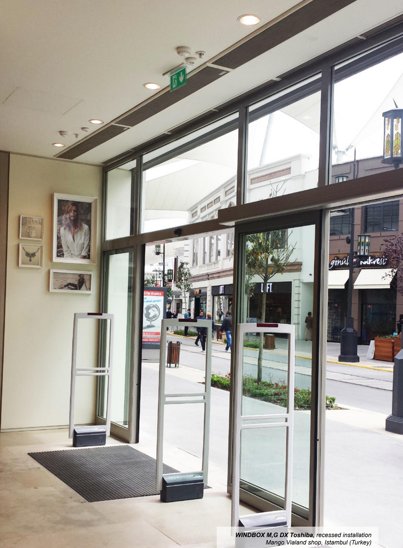
**WINDBOX M,G DX Toshiba**, recessed installation
