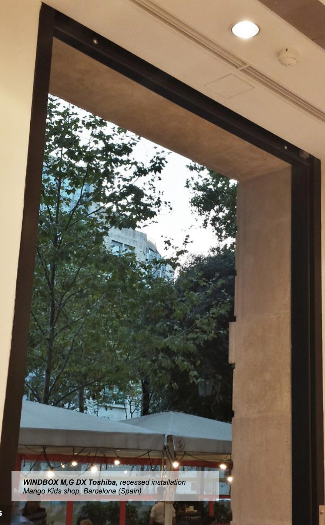
**WINDBOX M,G DX Toshiba**, recessed installation
