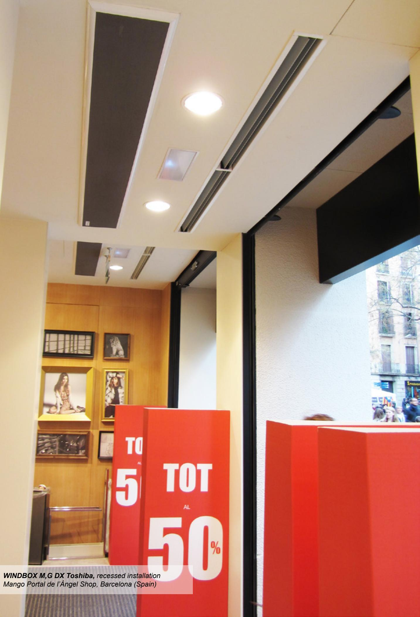
**WINDBOX M,G DX Toshiba**, recessed installation
