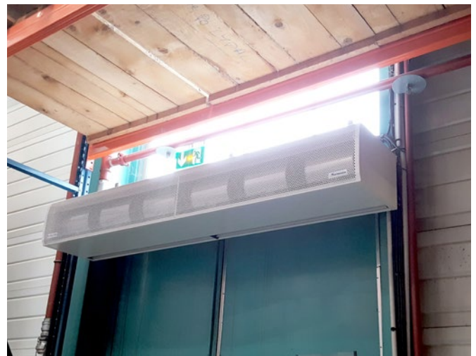
Fly KBB Installation in a packaging factory entranceway
