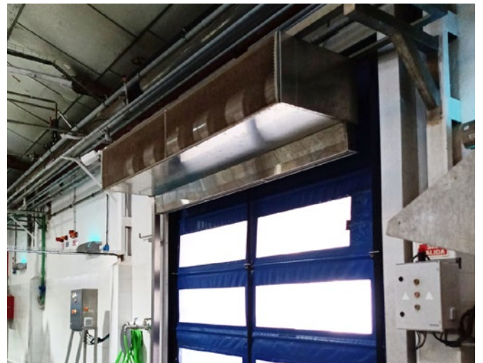
Fly KXL Installation in an anchovy and sardine factory
