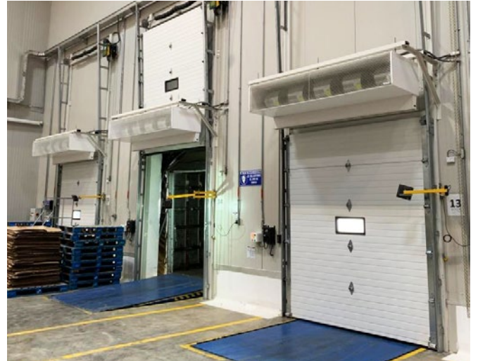
Fly KXL Installation in a food industry factory
