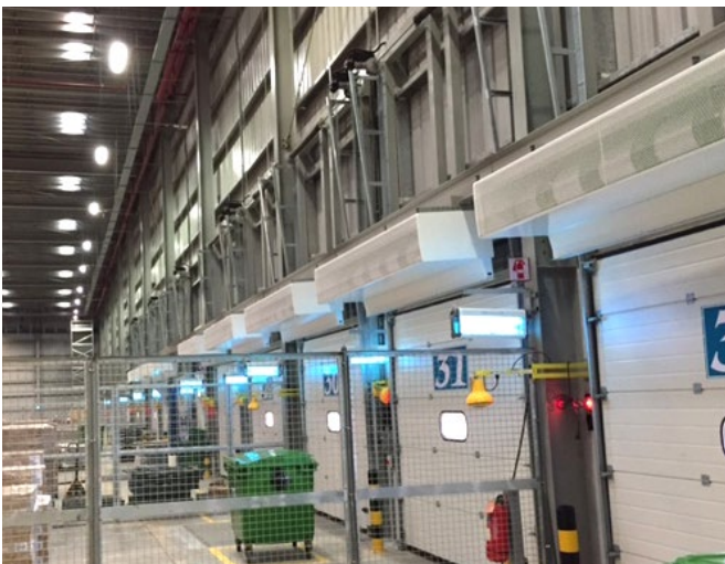
Fly KXL Multiple installation in a cosmetics and soaps factory
