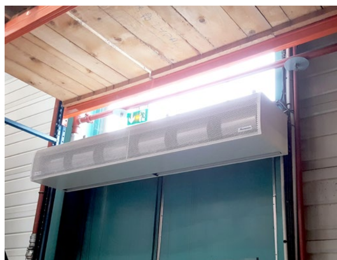
Fly KBB Installation in a packaging factory entranceway
